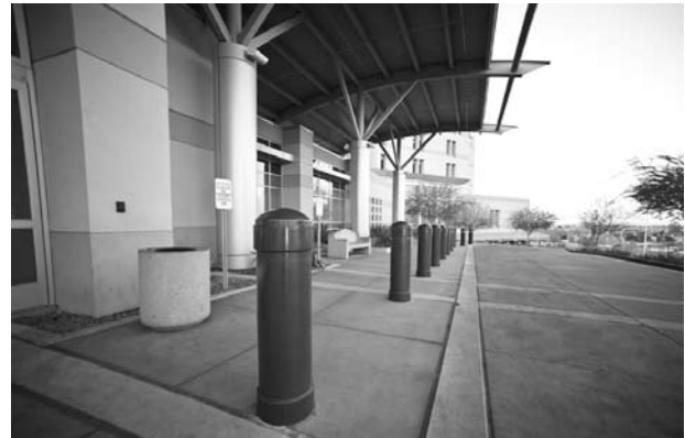
Rows of crash-resistant bollards protect entrances, glass areas, and main building of Yuma Regional Medical Center, Yuma, AZ. Reliance Foundry Co. Photo
