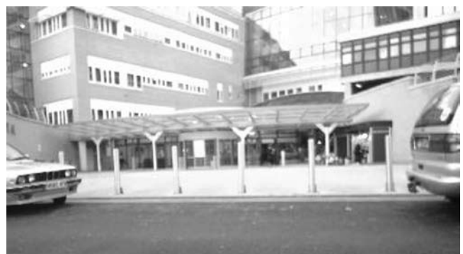
Street-located Whittington Hospital, North London, UK, has bollards at regular intervals to prevent passing vehicles from accessing the pavement.
